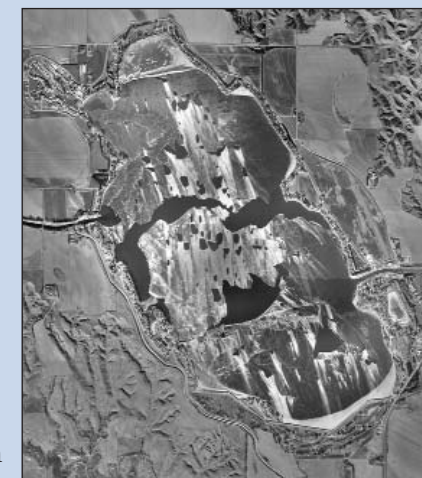
December 2003 aerial view of Johnson Lake
